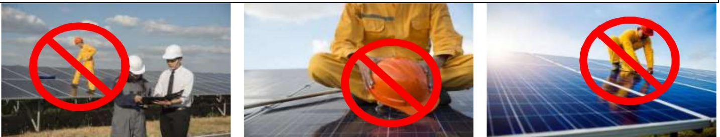
Wrong methods of installing a solar PV module
